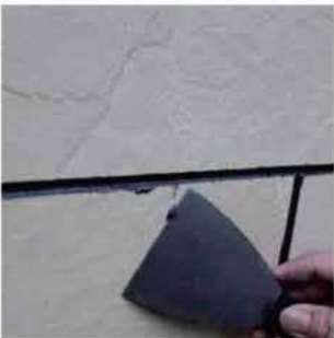
7. Use a hook to scrape off the areas contaminated by adhesive and cement slurry
