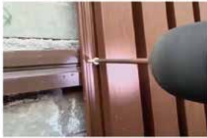
◦ Step 2 Secure the product to the studs.
