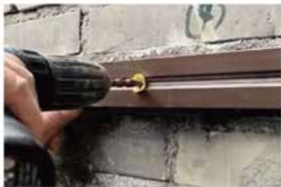
◦ Step 1 Fix the studs to the wall.
