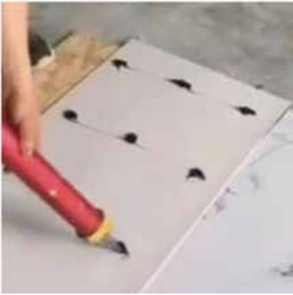
2. Apply glue to the back.
