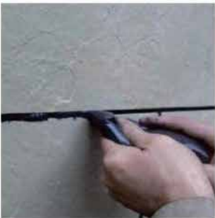
5. Use a plastic bag to fill the gap with grout or fill the gap with neutral silicone glue
