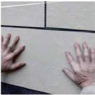
4. Move up and down to adjust the width of the space, and use a large board to compact the product to the wall
