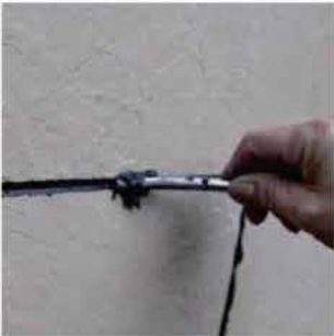
6. When the grout is half dry, use a steel bar to pull the seam
